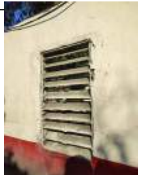
EXISTING LOUVER WINDOW TO BE REMOVED AND FILLED WITH CONCRETE, CEMENT PLASTER AND PAINT FINISH (COLOR: TO ARCHITECT'S APPROVAL)
